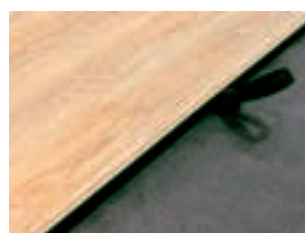
3. PRESSING INTO PLACE
