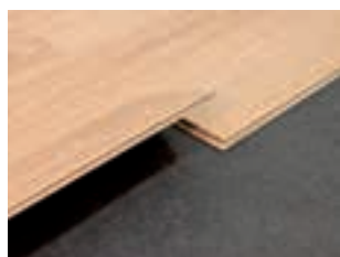
2. PRESSING INTO PLACE
