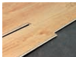
3. PRESSING INTO PLACE
